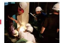
Damage observation in structural tests
